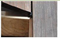
Angle the next board onto the partially screwed clip. Complete the row.
