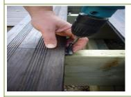
Clips should be level – do not over tighten.
