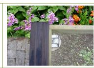
Place first plank (header board) on most obvious corner to start. Let the board hang over the frame a bit to trim later.
