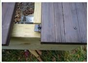
At header board, insert a clip in slot and partially drive screw until it just touches top of clip.
