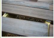
Double deck clips should be used at board seams. Single deck clips where there are no board seams.
